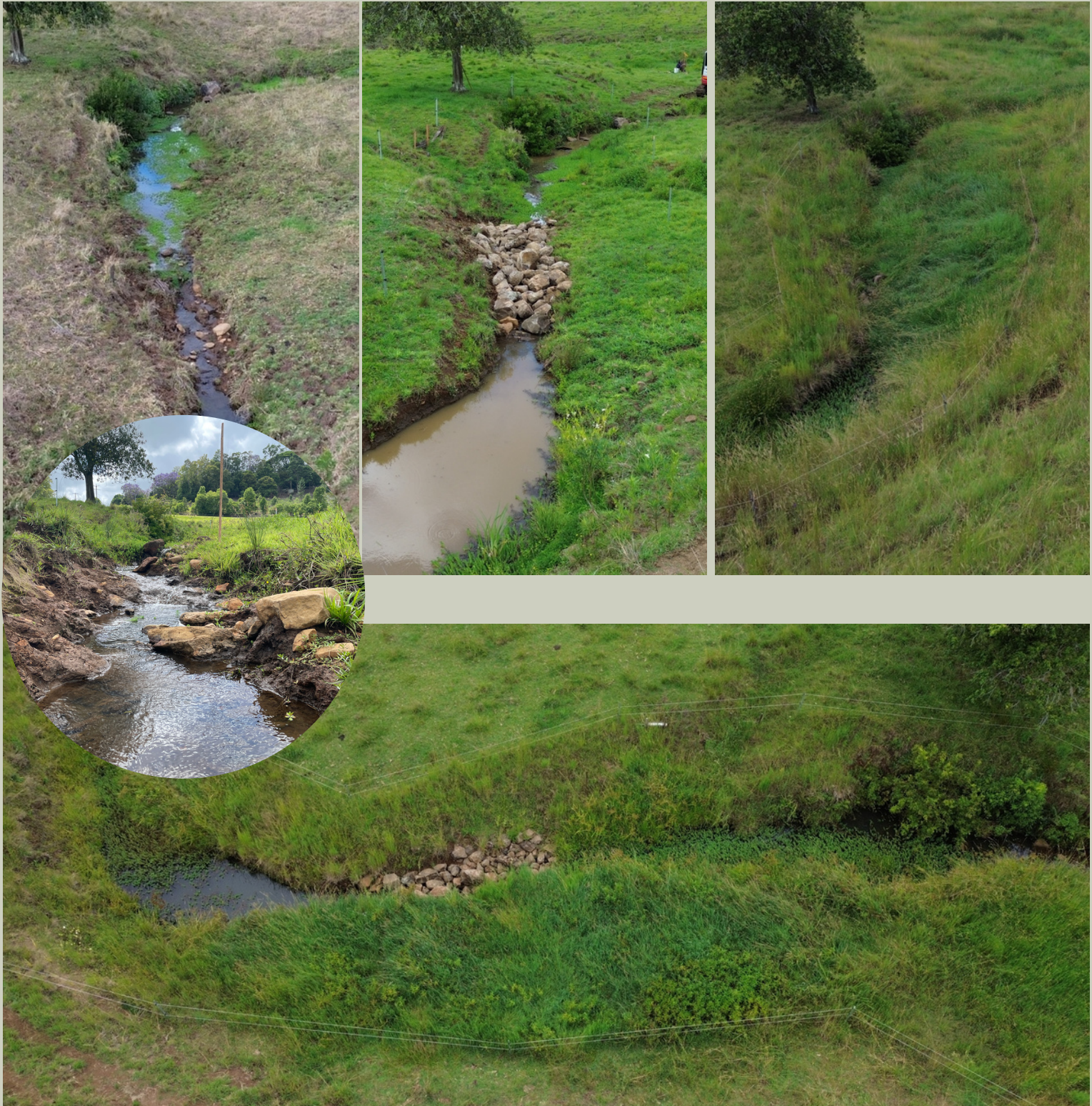
Placement of rock from site, planting and stock exclusion fencing.
